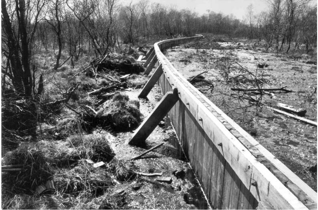
Figure 1 Pallisade timber dam lining compartment 2 in early spring 2002. Photo: Wilco Verberk
